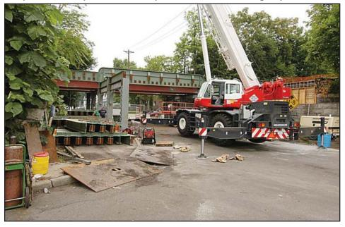
Steel erection for the NJ Transit bridge rehab in Plainfield. Final work required intensive historic replication.
